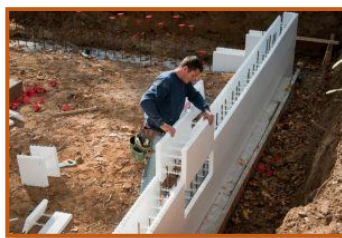
Fig: 14.10 Insulating Concrete Formwork (ICF) Technique
