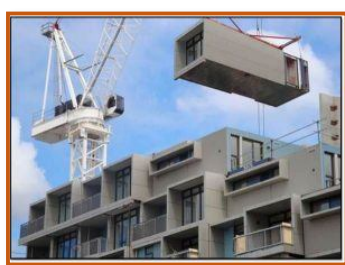
Fig: 14.3 3D volumetric Constructions
