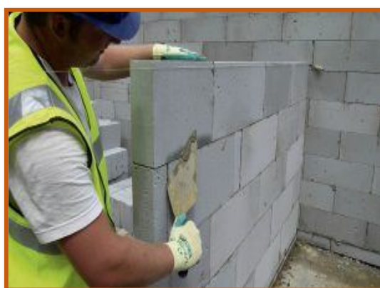
Fig: 14.9 Thin Joint Masonry Technique
