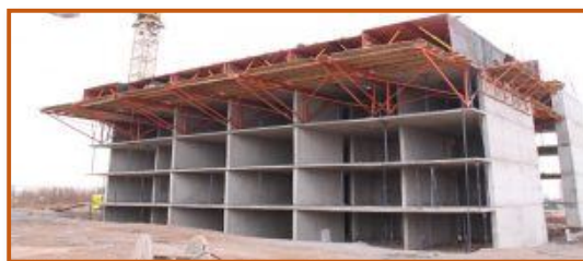
Fig: 14.5 Tunnel Formwork System
